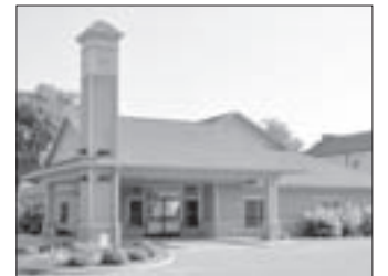
Office and Chapel 1501 West Avenue S., La Crosse
